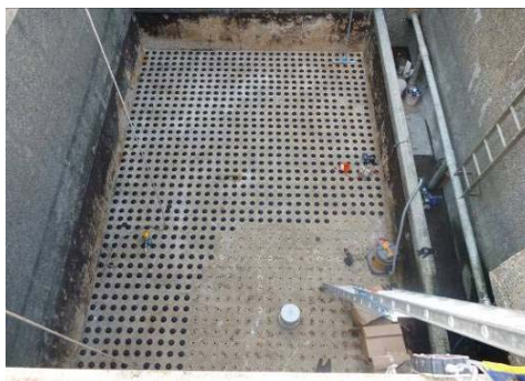
Figure 4: Nozzle installation
