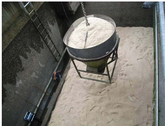
Figure 5: Installing media sand
