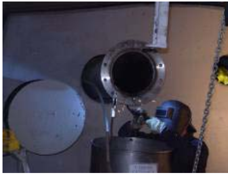
Figure 10: Welding table flange in place
