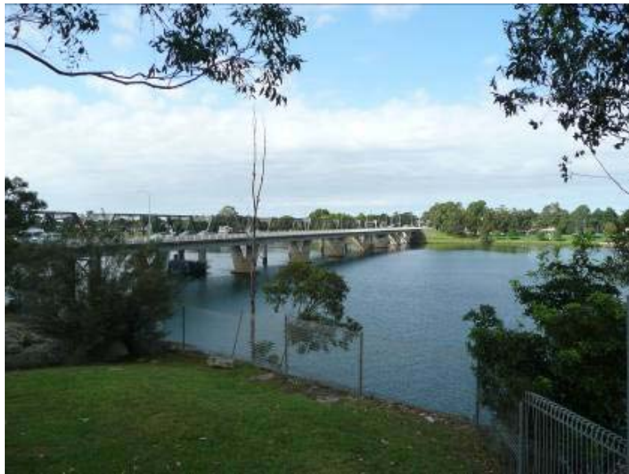
Figure 1: Shoalhaven River bridge
