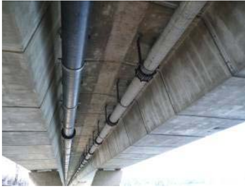
Figure 2: 300mm AC main on right
