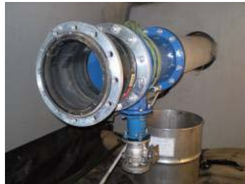
Figure 11: New expansion joint
