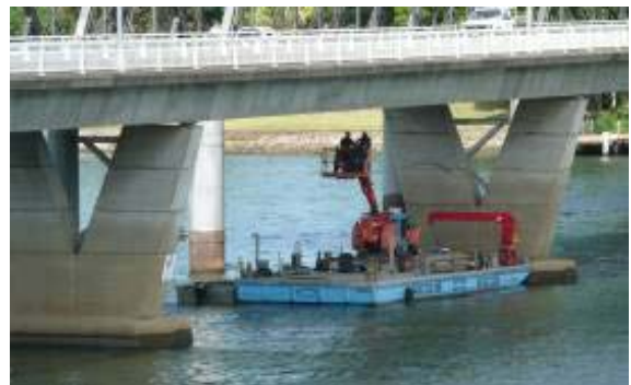
Figure 8: Positioning barge
