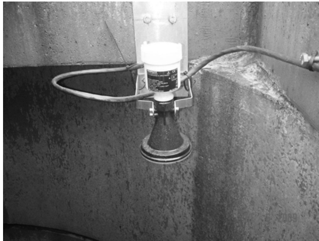
Figure 3: Installed radar sensor without touching the product
