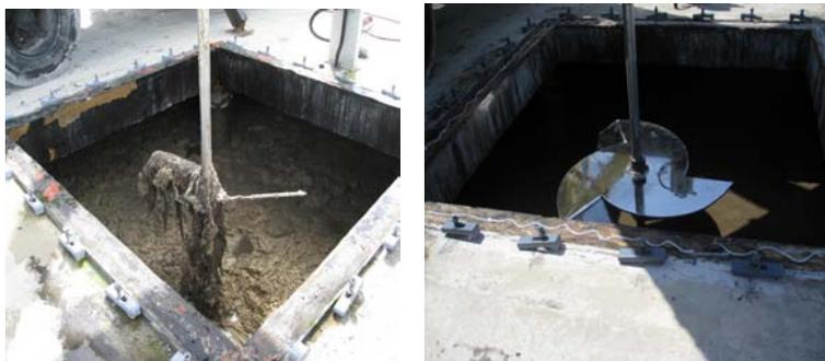
**Figures 4 & 5:** *The first Clean-Edge impeller installed in STP in USA*
