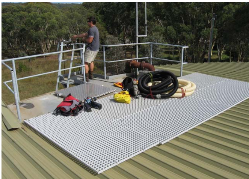
Figure 6: An upgraded platform area including additional guard rails.
