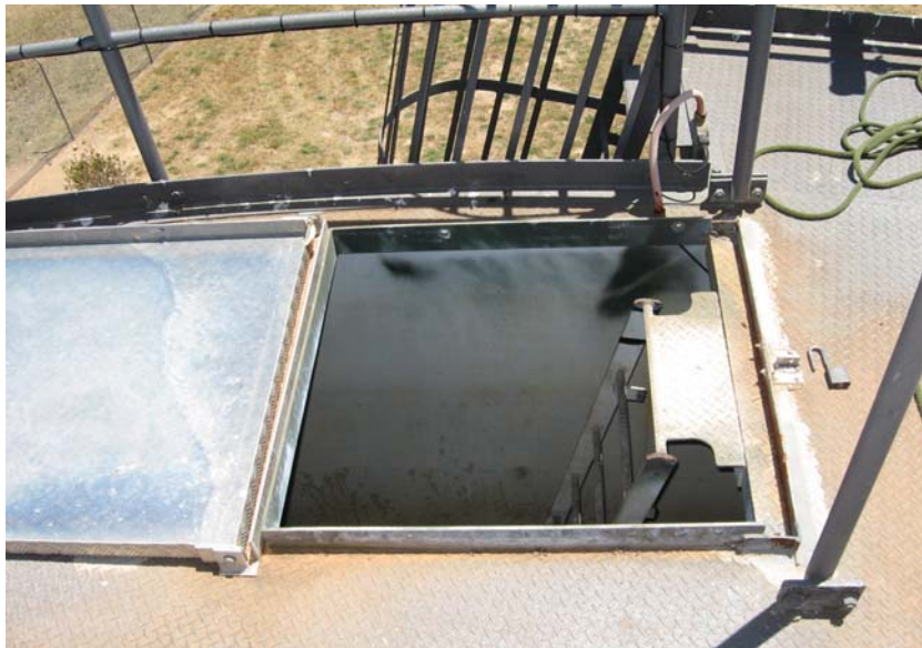
Figure 4: The existing ladder stiles trimmed off, the front edge sealed and an overlapping cover fitted.
