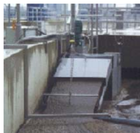
Figure 5: German developed scum harvester showing inclined belt drawing up scum to collection hopper.
