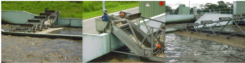
Figure 4: Biological foam harvester developed by APE showing dewatering beach with discharge hopper and collection buckets with scum baffle behind.
