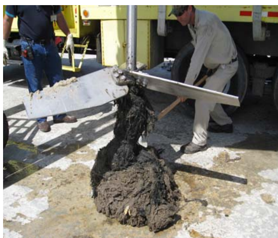
Figure 2: Clearing the impeller
