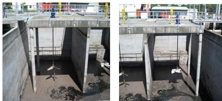
Figures 6 & 7: The new impellers at the Banora Point plant
