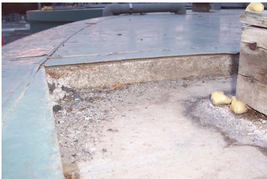
Figure 3: Foam insulation on ATAD tank
