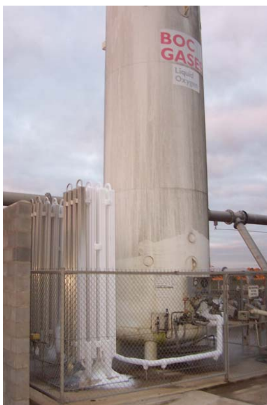
Figure 5: Cryogenic oxygen pressure vessel
