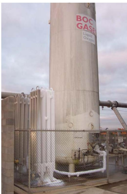
**Figure 5:** Cryogenic oxygen pressure vessel
