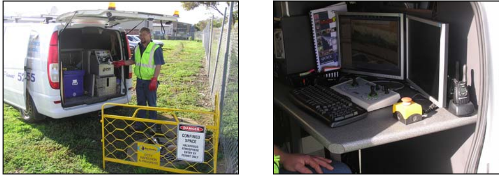
Figure 2: Camera van and on board control room showing dosing switch
