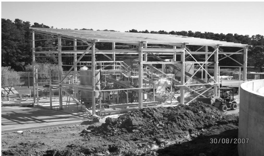
Figure 1: Thermal Dryer during construction
