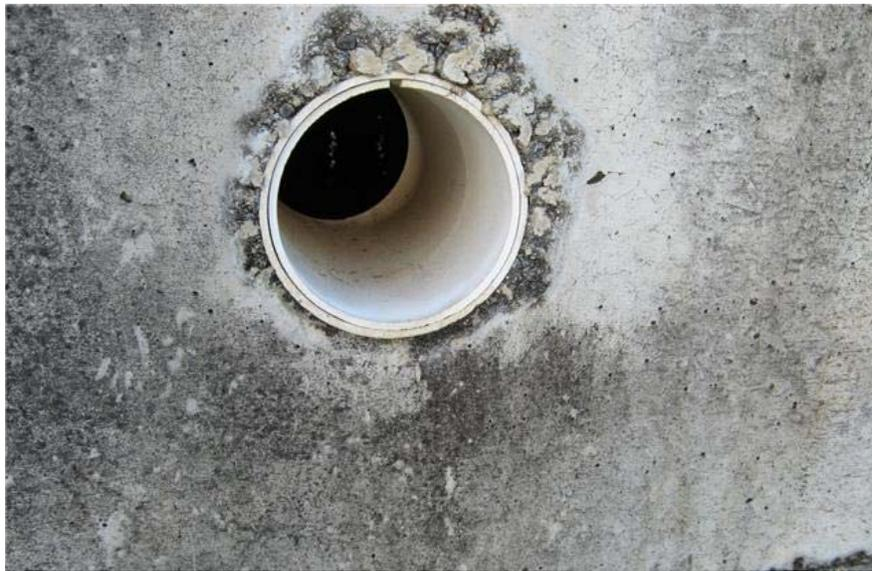
**Figure 1:** *An unsealed ventilation hole in the upper wall of a reservoir*
