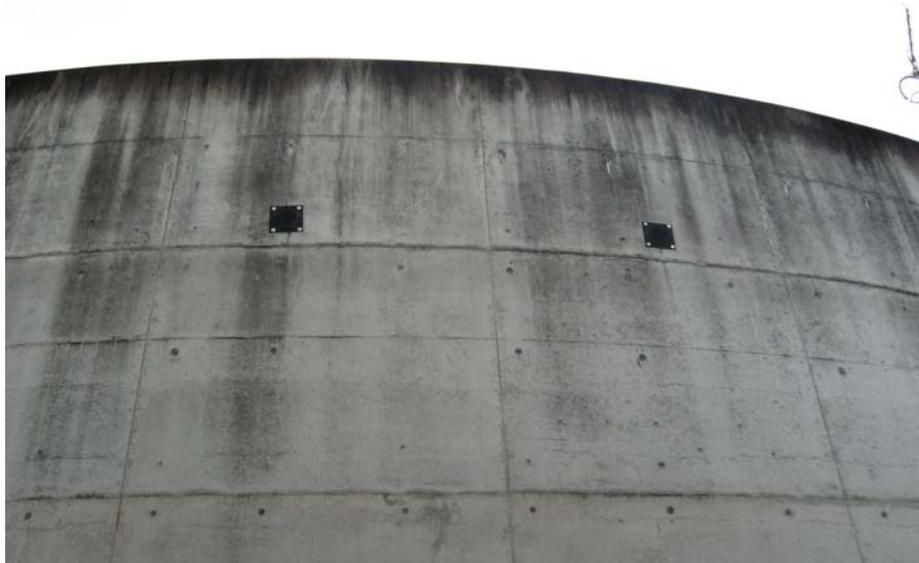
**Figure 6:** *The finished product; mesh screens secured externally over the ventilation holes*
