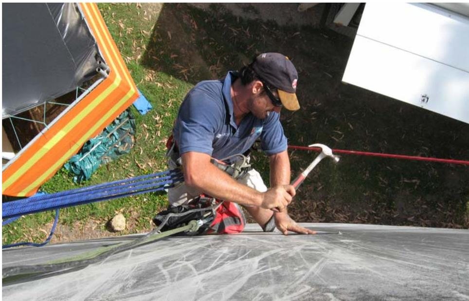
**Figure 4:** *The operator is held in position by a side rope from his harness (on right near hammer) leaving his hands free to complete his works effectively*
