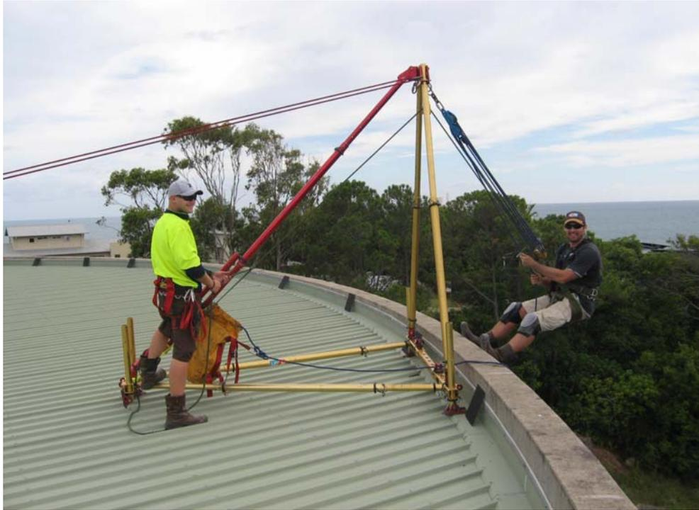
**Figure 3:** *Utilising the Oz Pod and advanced roping techniques to assess the upper walls of a reservoir*
