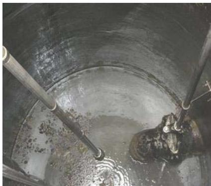
**Figure 2:** *Pump Station 14 days after installation of well washer*
