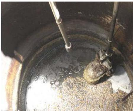
**Figure 1:** *Pump Station prior to installation of well washer*
