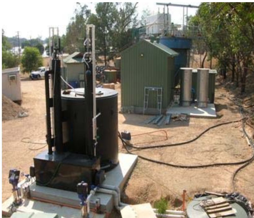
Figure 4: Progress on the upgrade of the Tarcutta WTP
