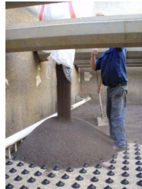
Figure 6: Rebuilding the Filter
