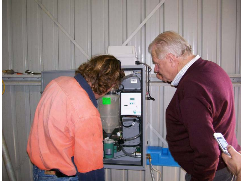
Figure 1: Chemsearch’s Peter Bennett explaining the operation of the Bioamp to Council Treatment Plant operator Marcus O’Reilly. The Bioamp installed inside inlet screen room at The Dru Point Wastewater lagoons 13/10/07
