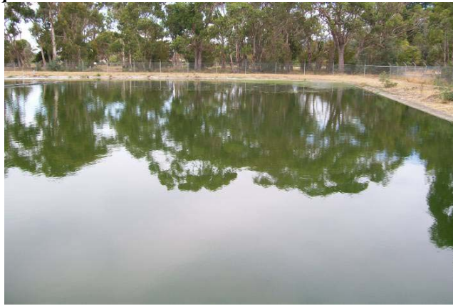
Figure 3: Top end of Primary Lagoon showing a marked improvement of lagoon with no floating sludge 4/02/08.
