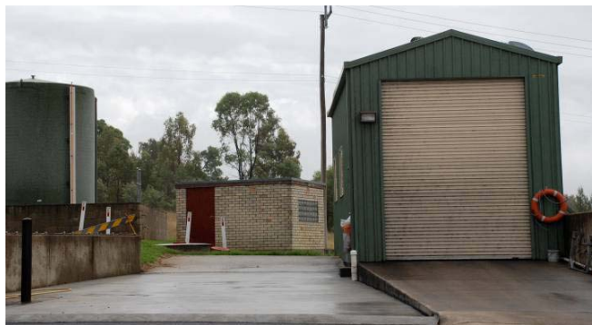
Figure 3: PAC Dosing Facility
