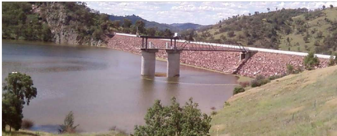
Figure 10: Chaffey Dam, Tamworth, spilling In November 2008.
