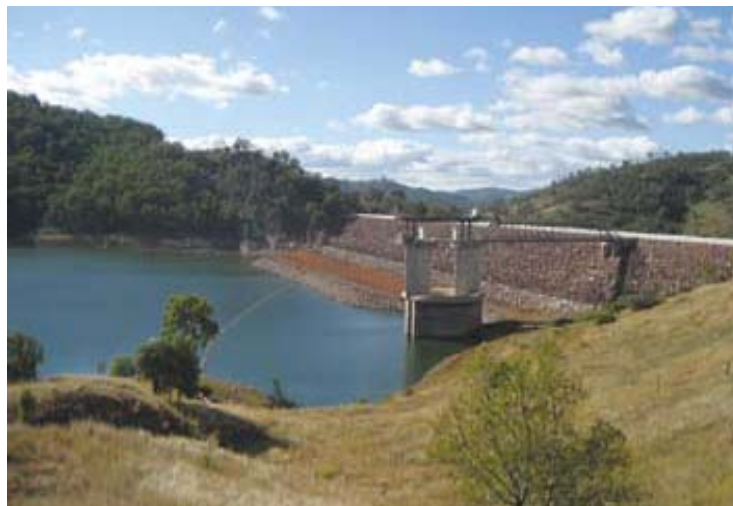
Figure 1: Chaffey Dam at 13.9% - March 2007
