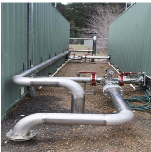
**Figure 3:** *Stainless steel pipework, fabricated and installed on-site*
