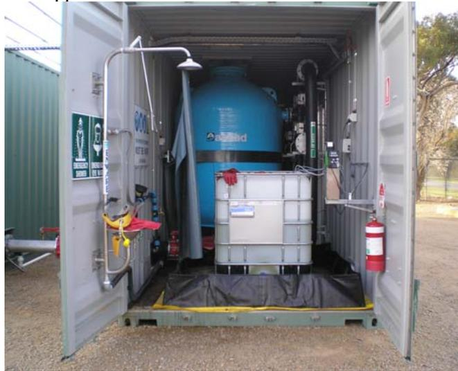
**Figure 1:** *Filter & chemical storage within a container*
