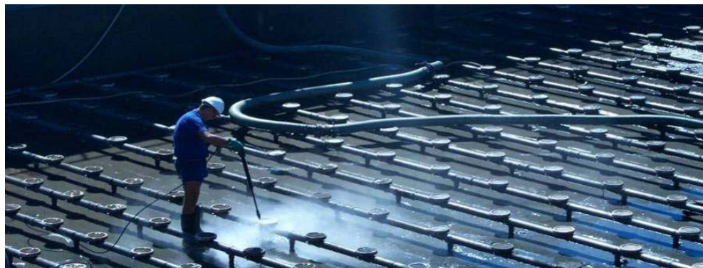
Figure 7: Diffusers being cleaned
