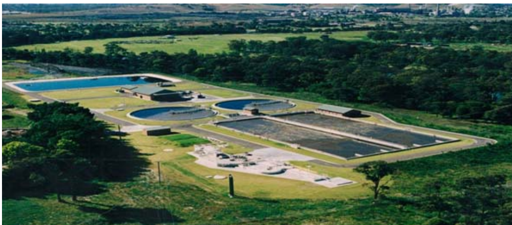
Figure 1: HWC's Edgeworth WWTW
