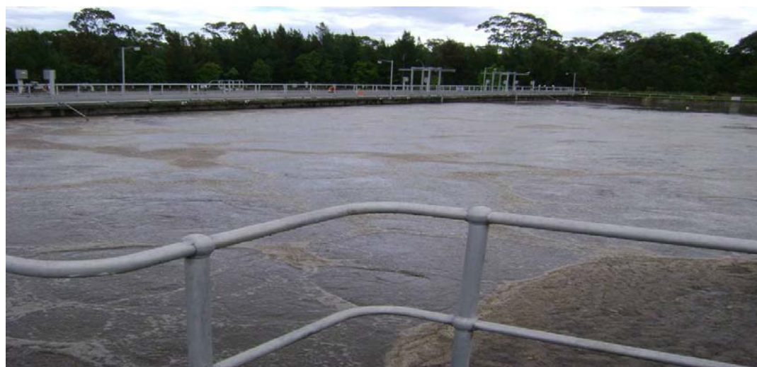
Figure 3: Bioreactor #2 at the Edgeworth WWTW
