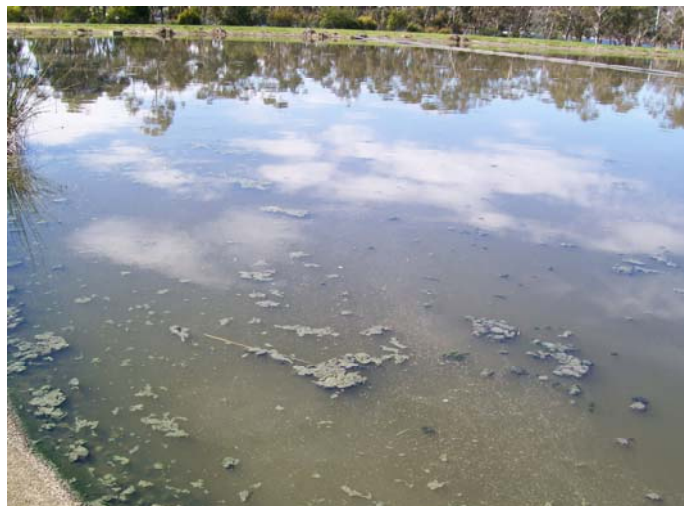
Figure 2: Top end of Primary Lagoon showing algae and floating sludge on day of installation of Bio Amp (13/10/07). This was indicative of all of the primary lagoon. The floating sludge and algae settled in the corners of the lagoon depending on the wind direction. This caused odour
