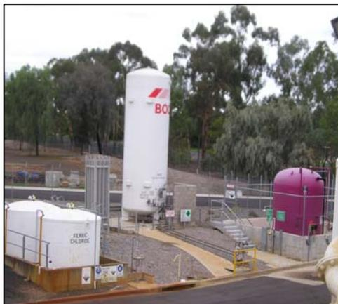
**Figure 4:** *New Ferric Chloride, carbon clearwater tanks*
