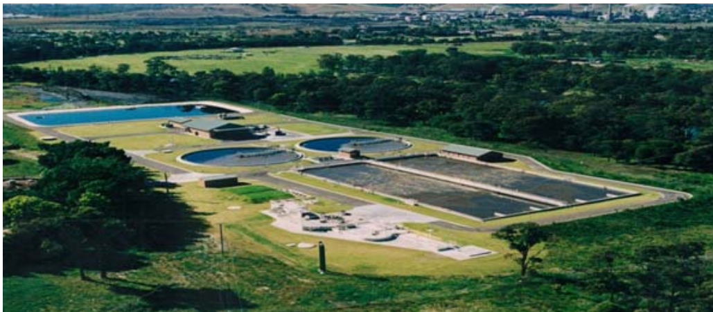
Figure 1: HWC's Edgeworth WWTW
