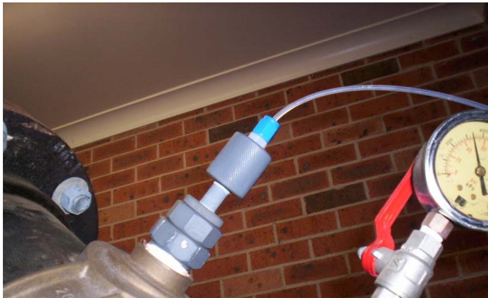
Figure 4: “Spearsafe” removeable injection spear
