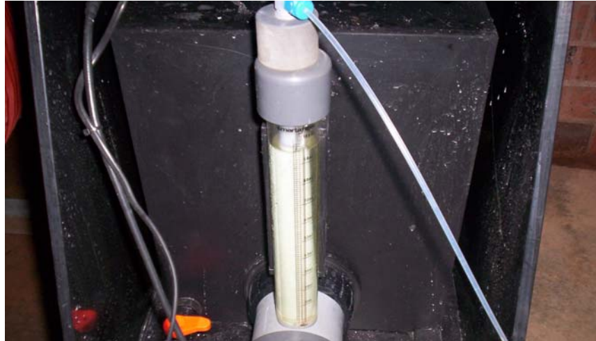
Figure 5: Smartaflow injection pump
