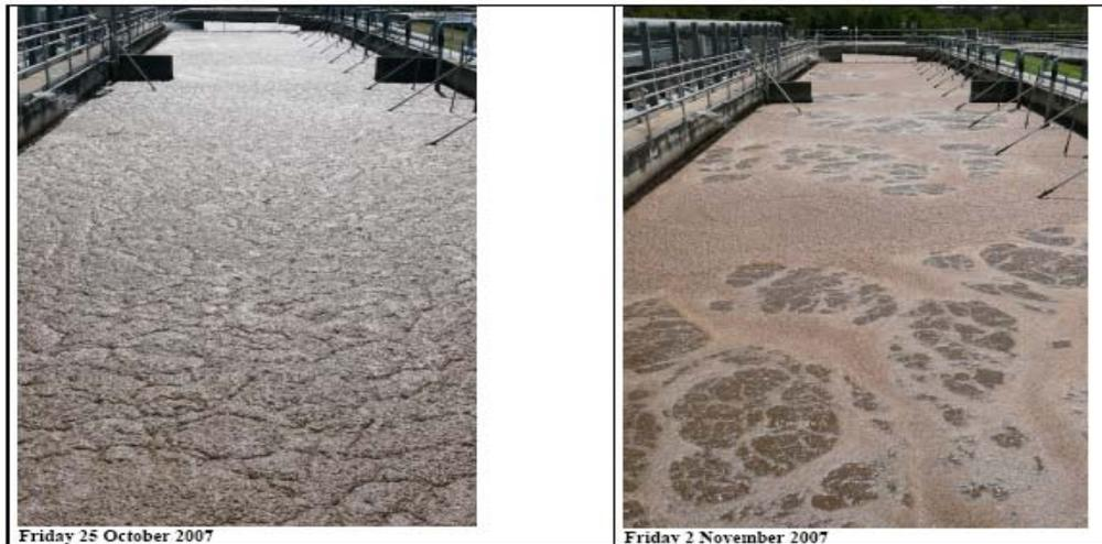
This trial ran for 4 weeks on Bioreactor 1. It was in the last two weeks we noticed that the ammonia and total N in the plant was reducing in the final effluent.
