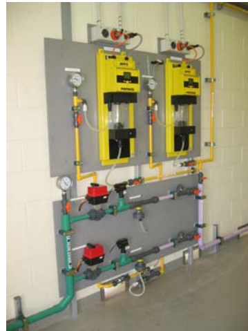
Figure 2: Typical duty/standby installation
