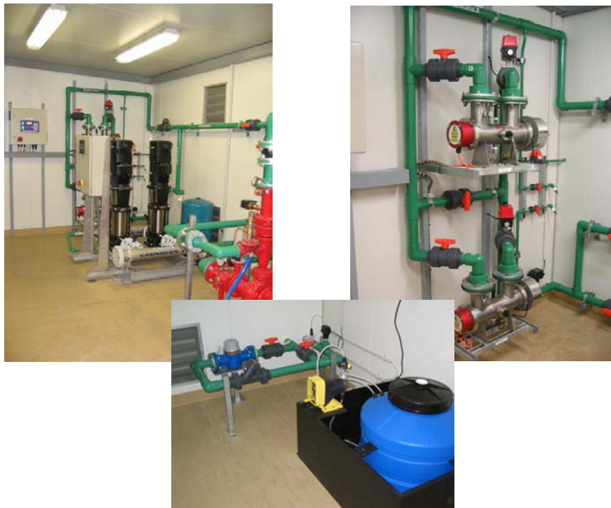
Figure 14: Potable water supply for a 350 man camp
