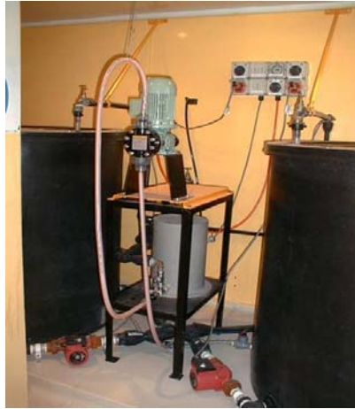
Figure 1: Things were upgraded
