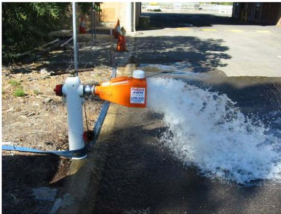
**Figure 7:** *Dechlorination Diffuser*
