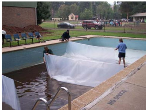
Figure 5: Temporary baffles in the Licola swimming pool.
