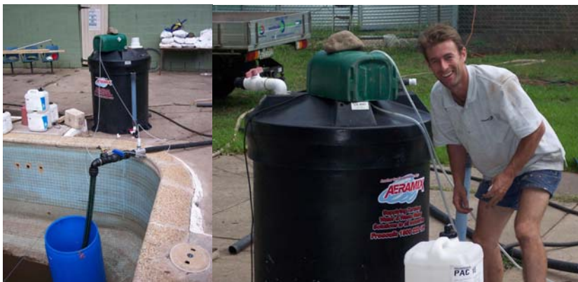
Figure 9: PAC mixing system and Jerry Rigged rapid mixing and diffuser tank.
