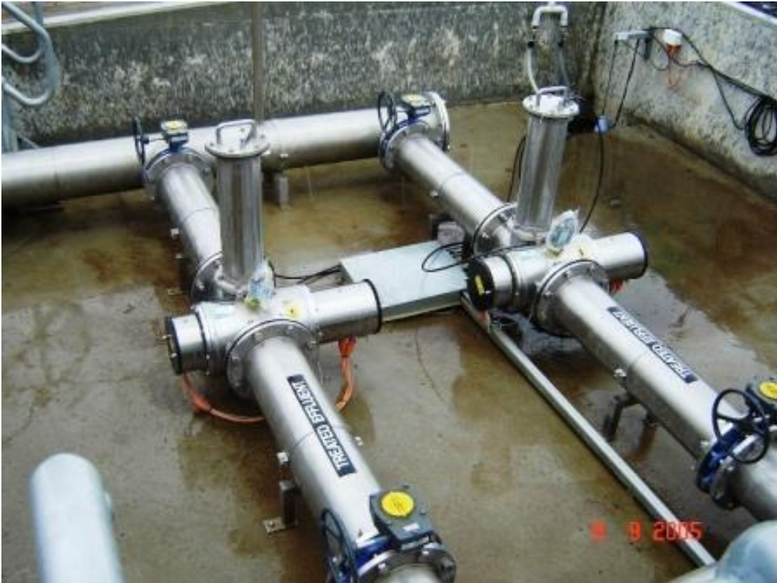
PHOTO SHOWS TYPICAL PARALLEL SYSTEM
