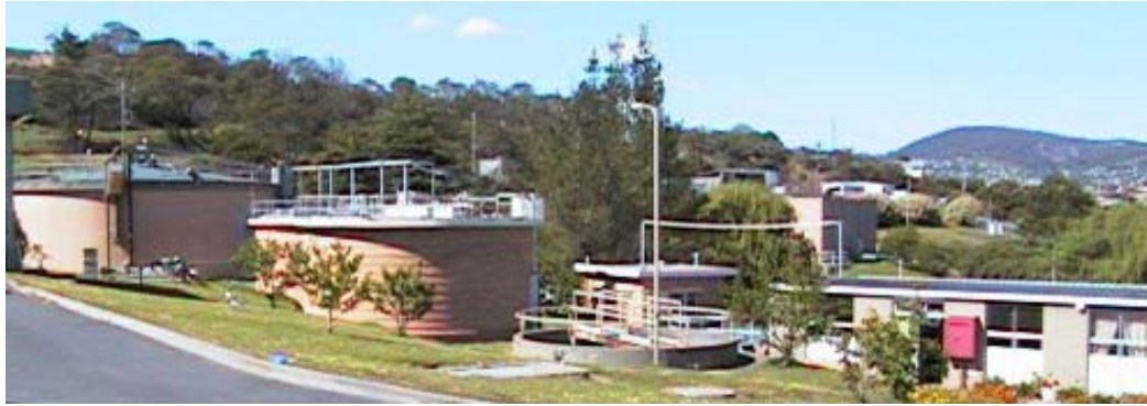
Figure 3: Glenorchy City Council STP (TAS)
