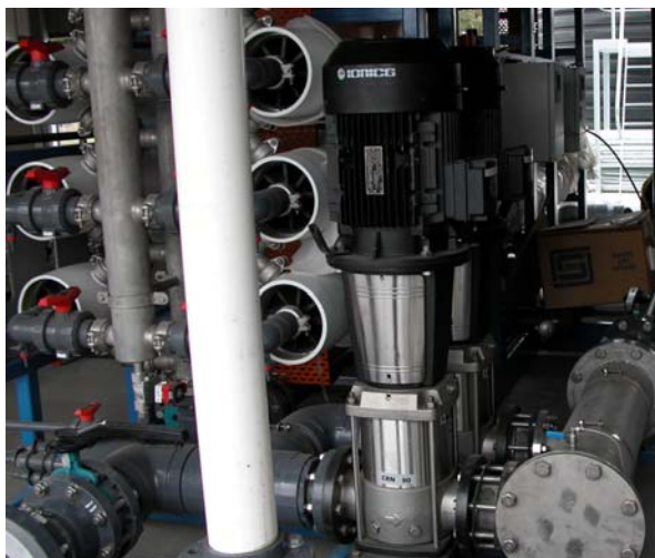
Figure 2: UF skid, with membrane modules shown
