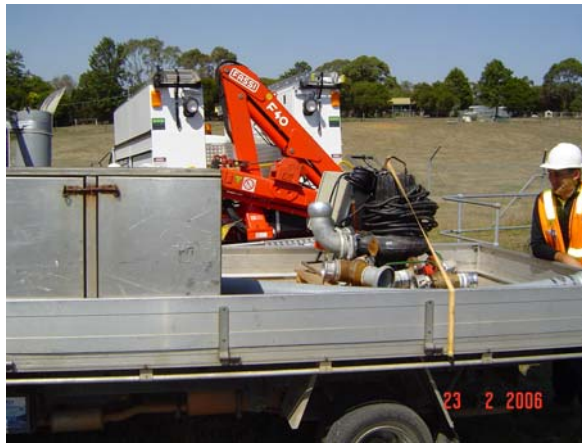
Figure 1: Submersible pump, switchboard and hoses loaded on a small truck.
