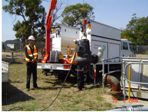
Figure 3: Unloading submersible pump with small crane truck.
