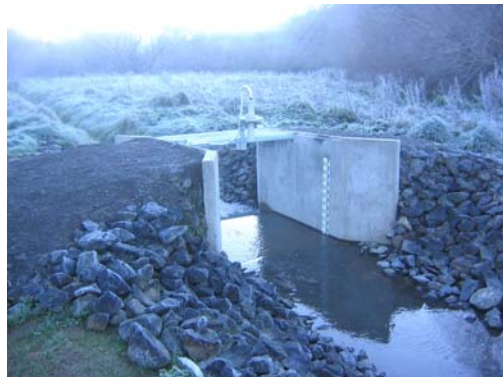
Streamflow Measuring, East Barwon
