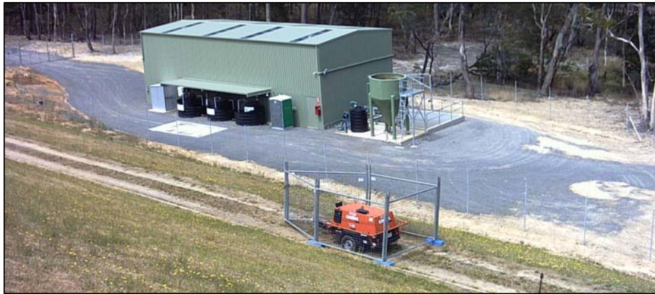
Figure 5: A Portable Air Compressor Installation At Musical Gully Reservoir
