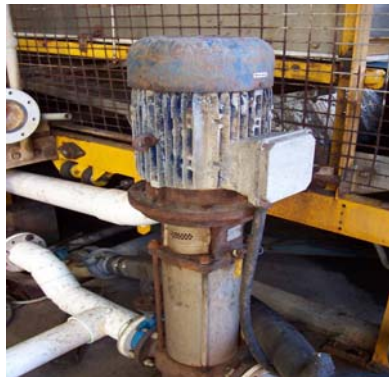
Figure 1: Corroded Wash Pump
