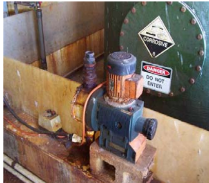
Figure 2: Corroded Ferric Dosing Pump
