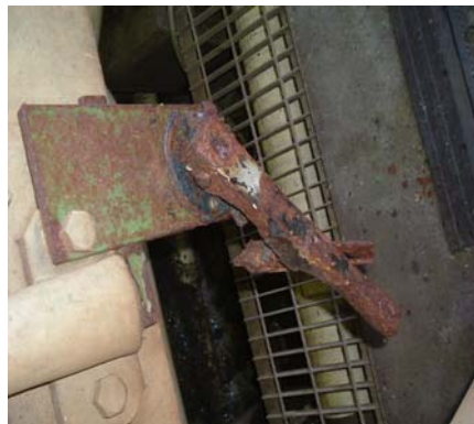
Figure 2: Corroded Ferric Dosing Pump
