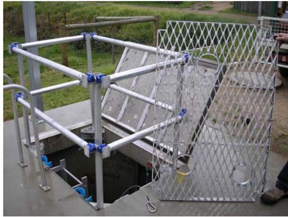
**Figure 4:** *Fully Installed Handrail System with Grate Removed*
