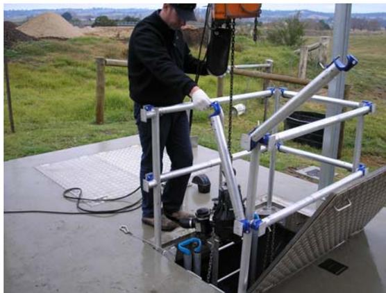
**Figure 5:** *Practical Use of the Handrail System – Removing Pump*
