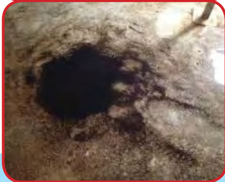
Dislodged particles inside treated water storage tank
